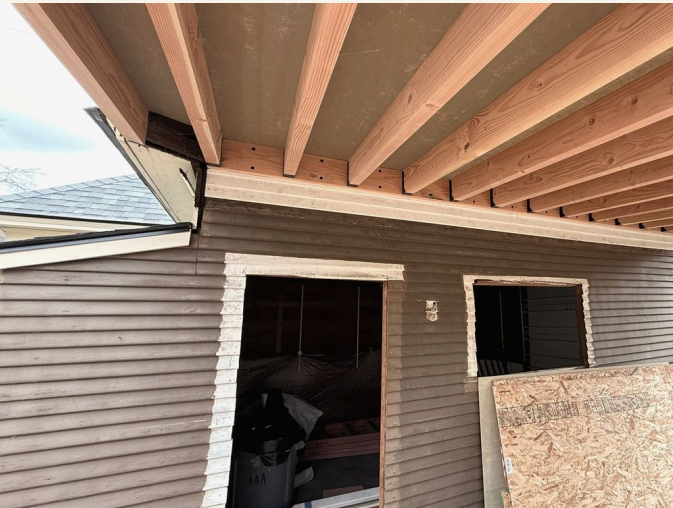
Mid-build, 18 February 2026 — the ledger taking hold of the existing house: the HUC 38 hangers from the roof-to-ledger detail, installed.
