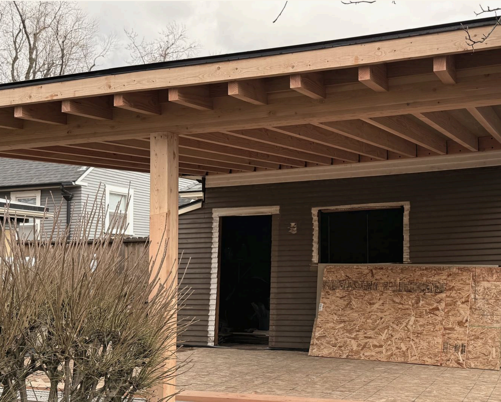
18 February 2026 — the structure framed, mid-build. Finished later that month.
