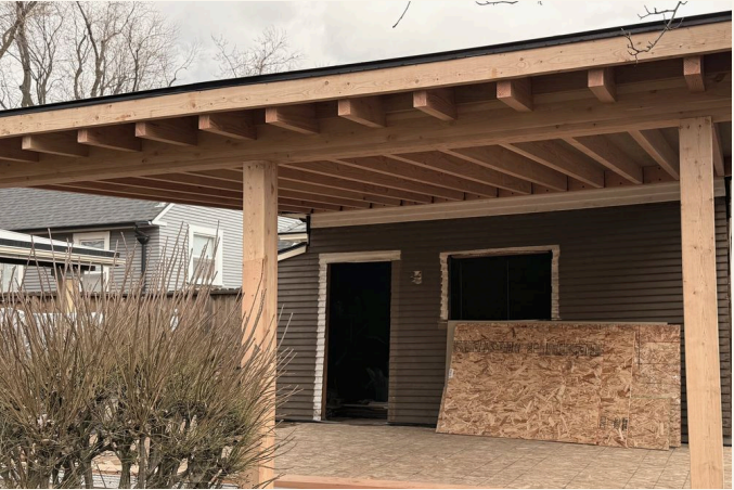
18 February 2026 — the structure standing, mid-build: the posts, the beam, and the rafter tails the details promised.
