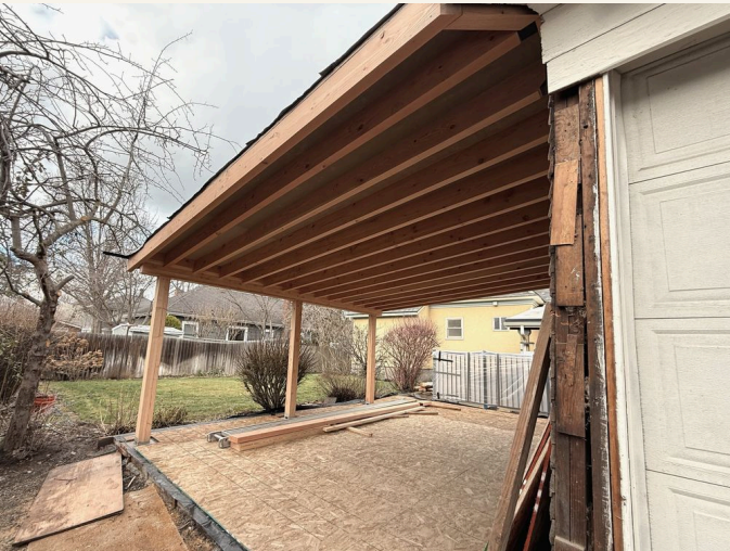
Mid-build, 18 February 2026 — standing under the drawing: the rafters at sixteen on center, exactly as the framing plan runs them.
